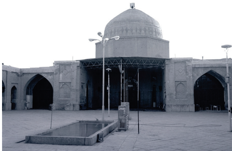
Fig. 4 Golpaygan, Great Mosque. Courtyard to SW (2008)
